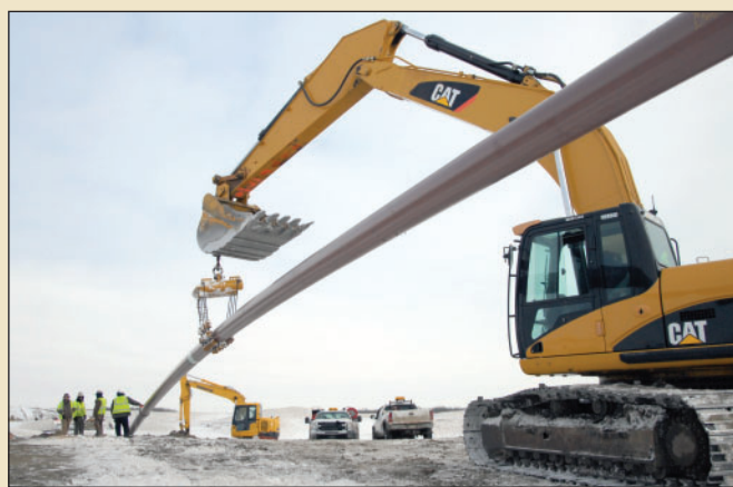
A roller cradle supports pipe in a horizontal drill pull-through during construction of Alliance's Tioga lateral pipeline.
