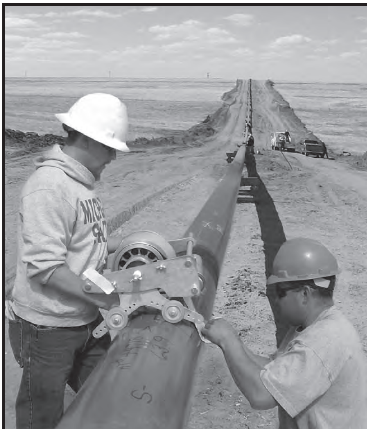
One of thousands of projects using Polyguard RD-6 non-shielding coating. Our first was in 1988.
