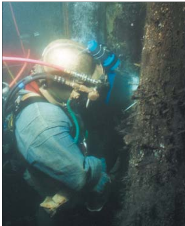
An American Marine Corp. diver welding an underwater dock structure
