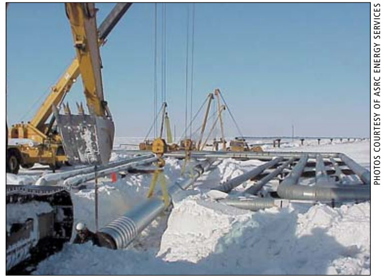
At left, fabricating the modules for the Alpine field at ASRC Energy Services' Nikiski facility. Above, Houston Contracting Co. laying the water injection pipeline L3 crossing for the GCWI project at Prudhoe Bay
