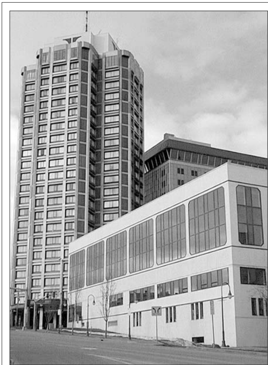
Alaska Anvil's offices, 509 W. Third Ave., Anchorage, Alaska
