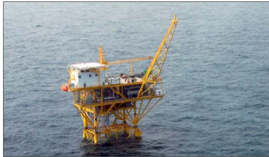
Pioneer, which has been steadily adding production from the Gulf of Mexico such as the Falcon platform pictured above, could see a second-quarter profit of 72 cents per share compared to 58 cents per share in this year's first quarter.
