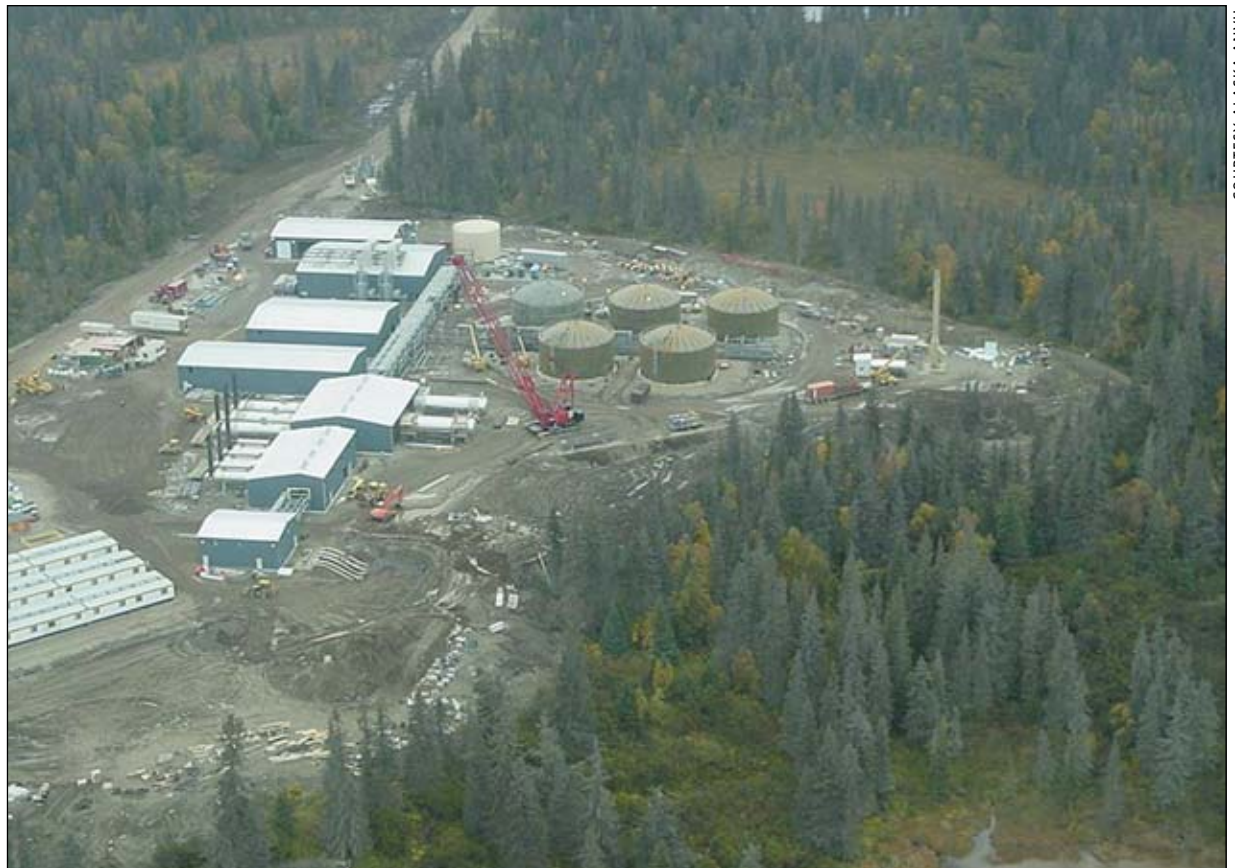
Cook Inlet production facility
