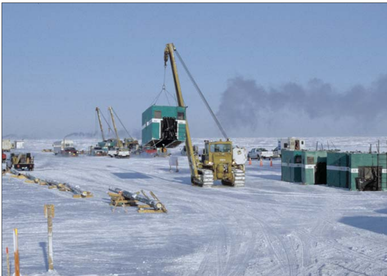
ASRC Northstar off-shore pipeline operations begin on the floating Beaufort Sea ice, with the pipe being strung out and the welding shacks put in place by sidebooms.
