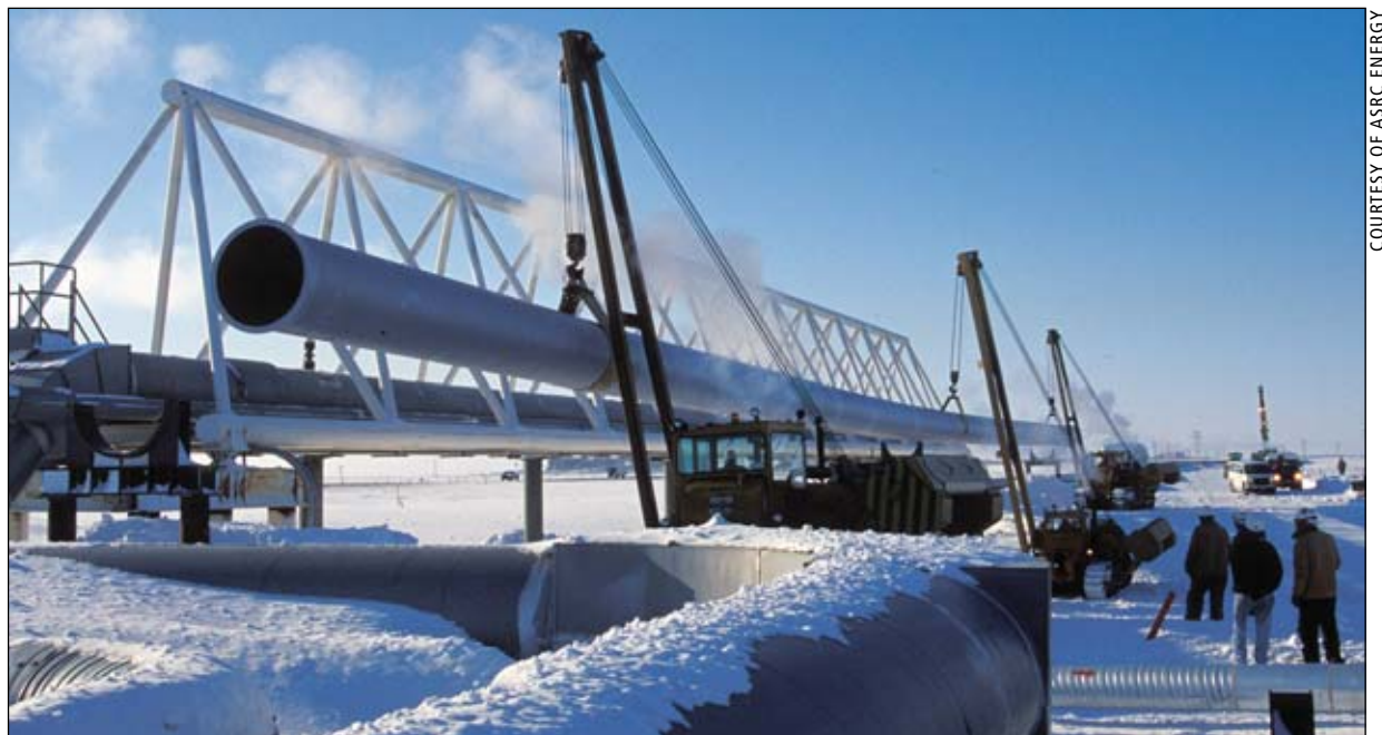
48" Pipe Bridge being installed across the Putt River to act as a carrier for the Northstar oil pipeline.
