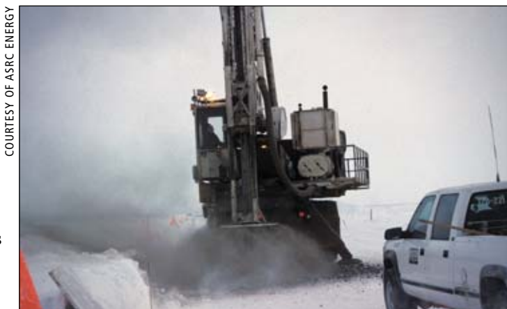
Watson 3000 Air Drill, drilling holes for vertical support member's installation for Northstar.
