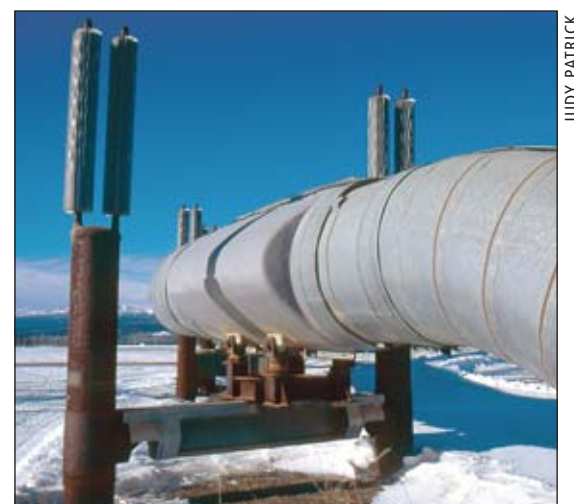
The 800 mile trans-Alaska oil pipeline runs from Prudhoe Bay to the Port of Valdez.
