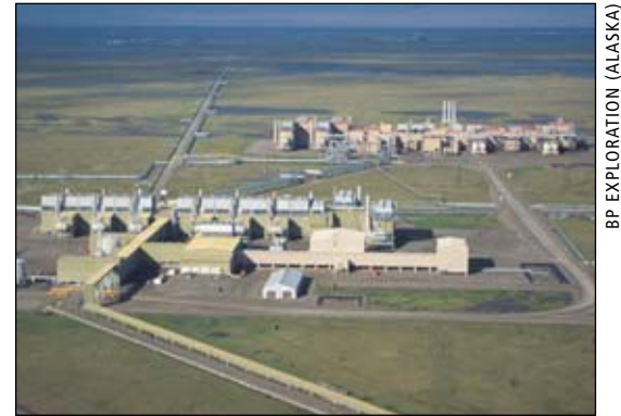
Pictured above is the Central Gas Facility at Prudhoe Bay where gas is largely re-injected back into the field.
