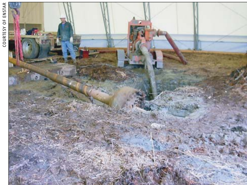
Fly-cutter reamer used to enlarge hole for natural gas transmission pipe
