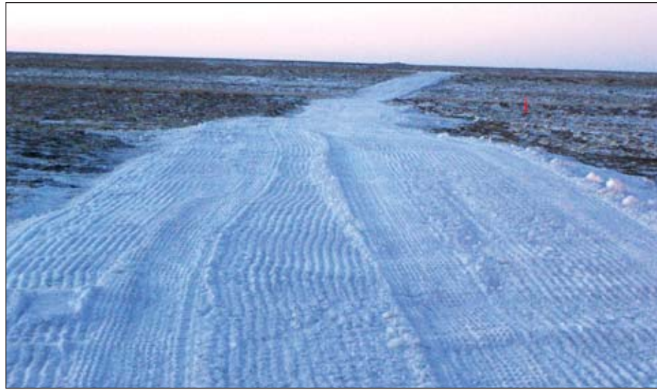
Pre-packing an ice-road route with snow and ice chips conserves snow, ready for road construction, as well as improving tundra protection.
