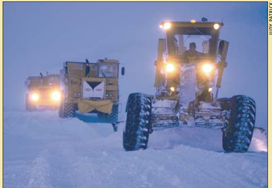
Building ice roads on Alaska's North Slope
