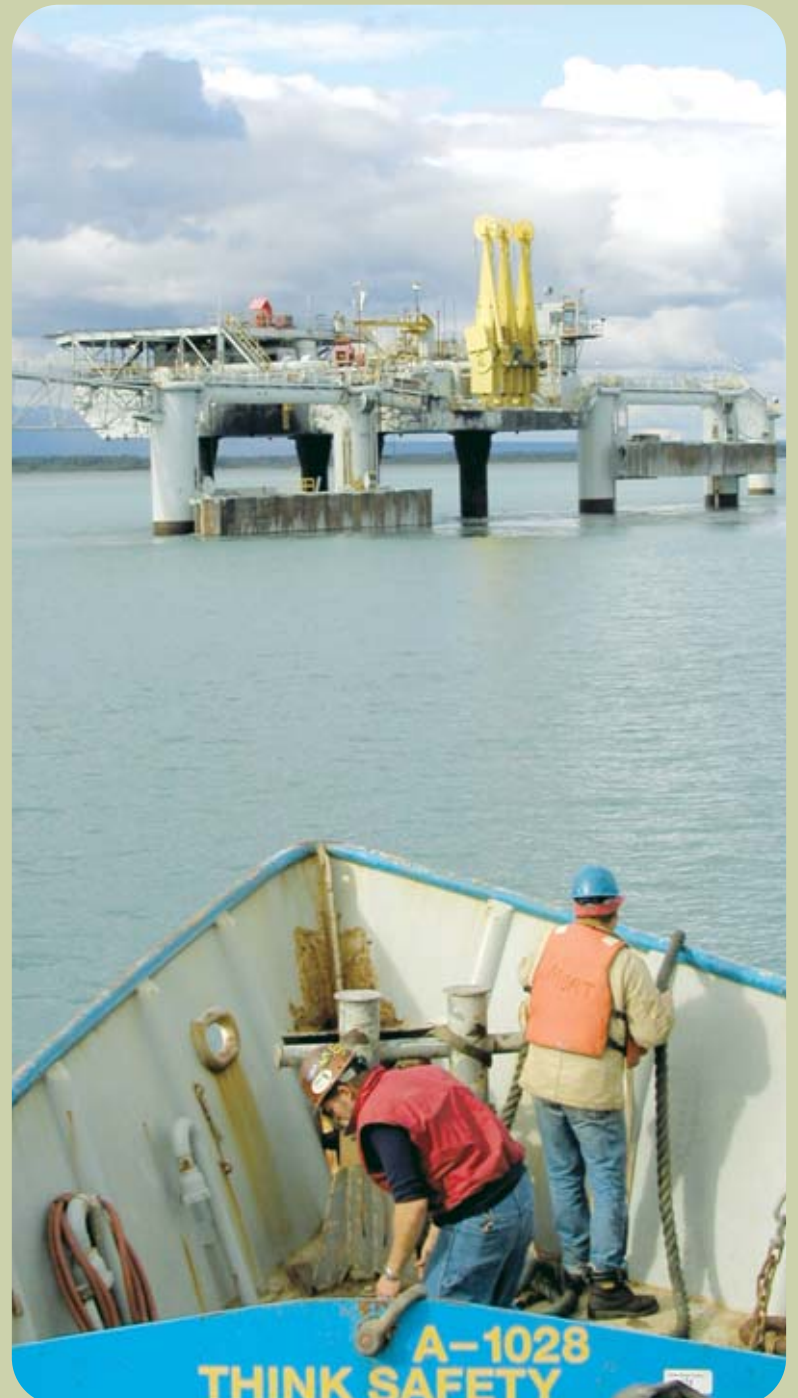
Christy loading platform in Cook Inlet
