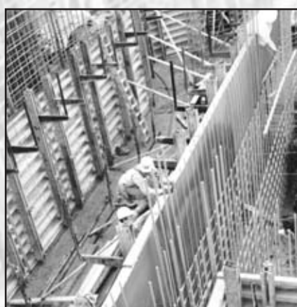
Bradley Lake Hydroelectric Project. Homer, Alaska
