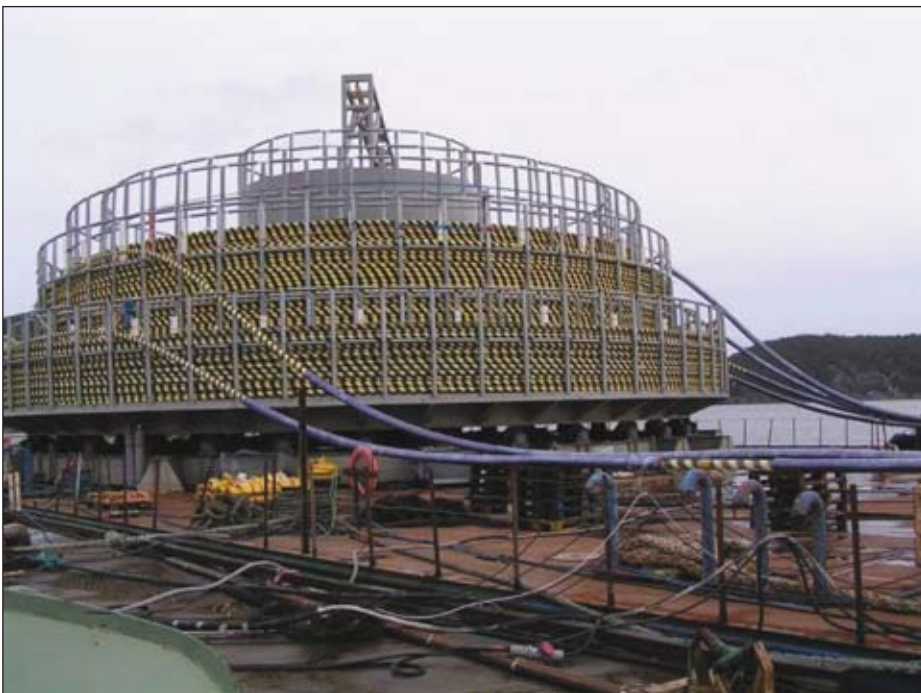
The main 89-mile-long umbilical for Snohvit was transported by barge.
