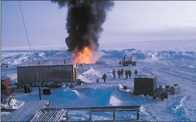
Drill stem test No. 5 on Feb. 18, 1968, recovered both gas and oil and clearly showed that oil could be produced from Prudhoe Bay State No. 1
