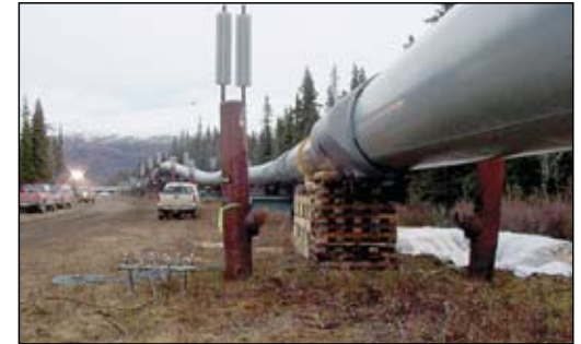
A 7.9 magnitude earthquake in November 2002 prompted a temporary shutdown of the trans-Alaska oil pipeline.
