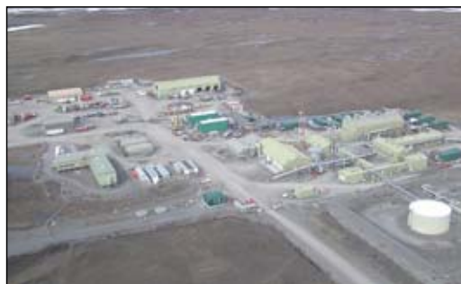
Pump Station 3, north of the Brooks Range (photo taken in June 2006). The dark green buildings are the new facilities. These include three variable frequency drive modules, three pump motor modules, and two turbine generator modules.
