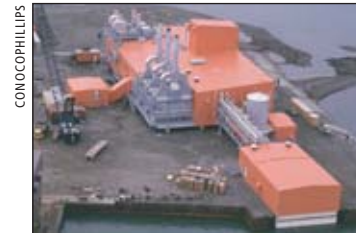
Seawater Treatment Plant Courtesy Conoco Phillips
