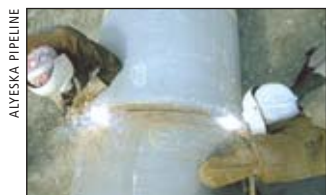
Final pipeline weld near Pump Station 3, May 31, 1977..
