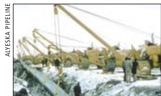
Pipe being laid at Tonsina River.
