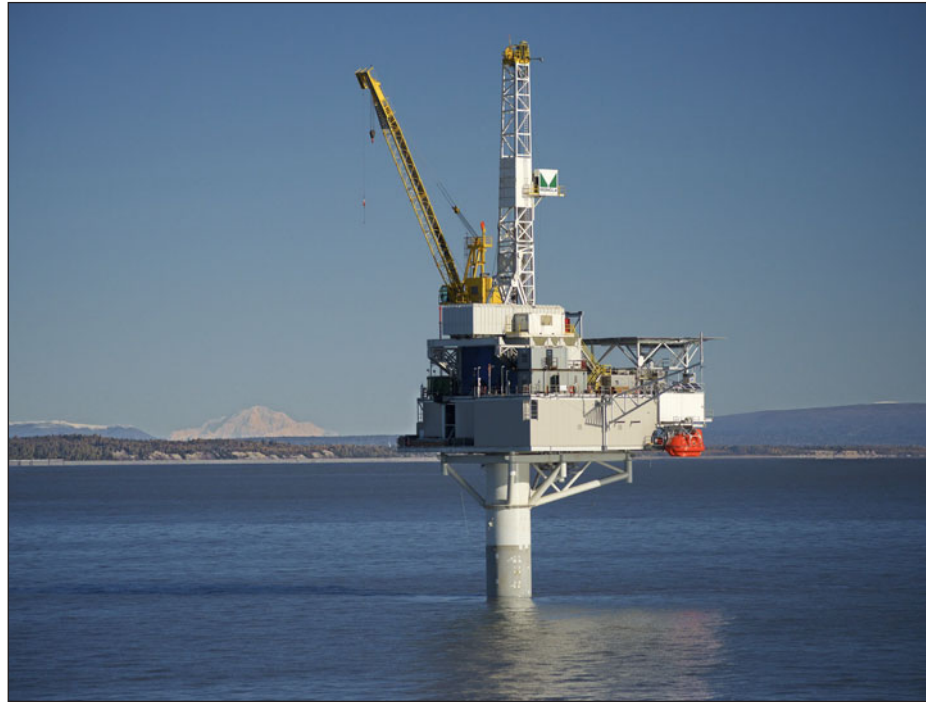
The Julius R platform offshore in the Cook Inlet produces gas from the Kitchen Lights field.
