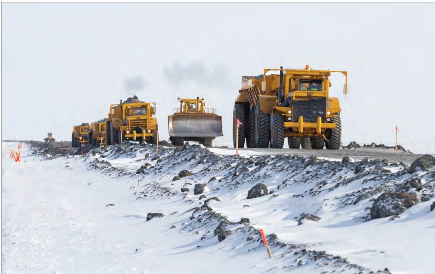
Western North Slope gravel road construction.
